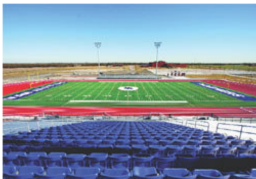
The high school synthetic field installation by Hellas Construction is the home of the Van Alstyne (Texas) Panthers.
